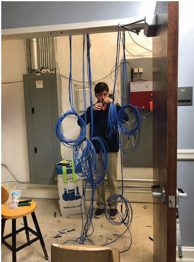
Jacob Holston '23 wires a building for improved technology.
